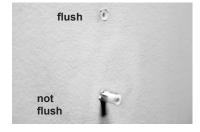
Remove  $\mathbf{K},$  drill and insert the second  $\mathbf{M}$  and hammer it until flush with the wall.
