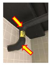
Photo 1: Asbestos-containing parging cement insulation on pipe elbows – Men's Washroom.
